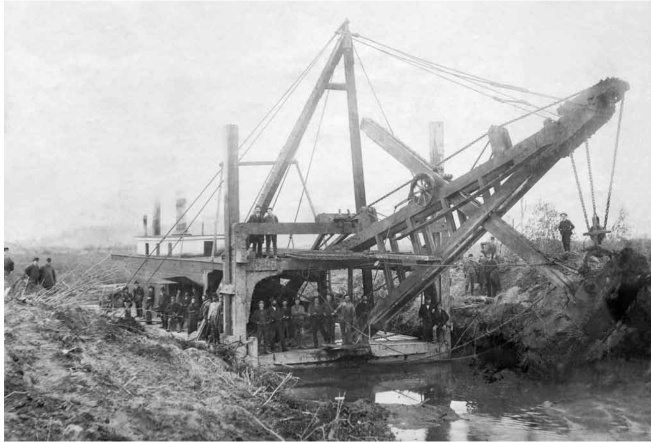
A floating dredge used in the attempted reclamation of the north Pitt Meadows around the turn of the century.
