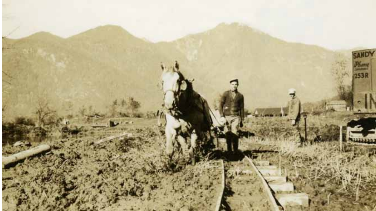
Lammert Westerhof's horse pulls a cart along a narrow-gauge track. The cart contained a cubic yard of building material that was dumped in order to build up the dike at the Deep Slough. The horses used in the project were an effective means of compacting the soil. 1951.
